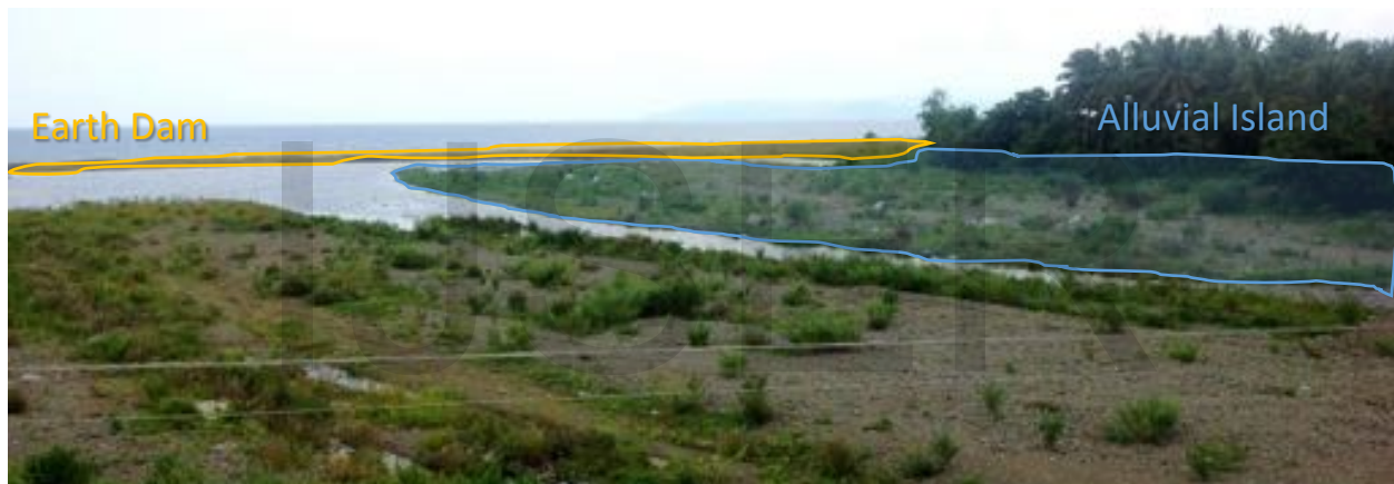
Figure 3.29 View looking S18°W taken at 15.28°N, 121.39°E showing the alluvial islands, active course of Dingalan River, and non-engineered earth dam composed of clay to fine sand materials.
