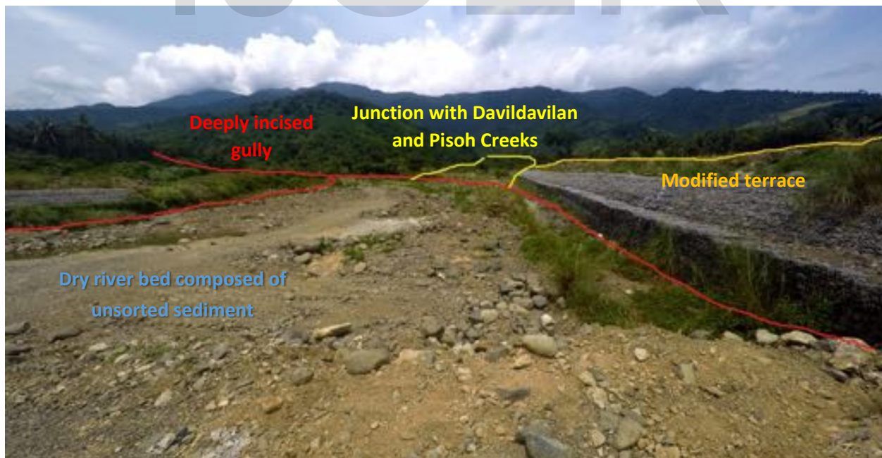
Figure 3.10 View upstream of the Langawan River with facing direction N35°E taken at 15.39° N, 121.39° E showing the dry river bed, location of the gully, and modified river terrace on the river banks.
